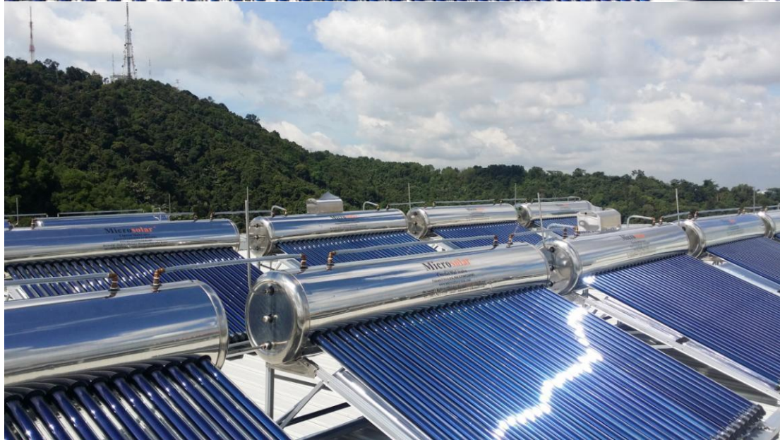
50 units Microsolar Water Heaters M80VTHE at University Campus and Hotel at Taman Connaught Cheras Kuala Lumpur Malaysia 2017
