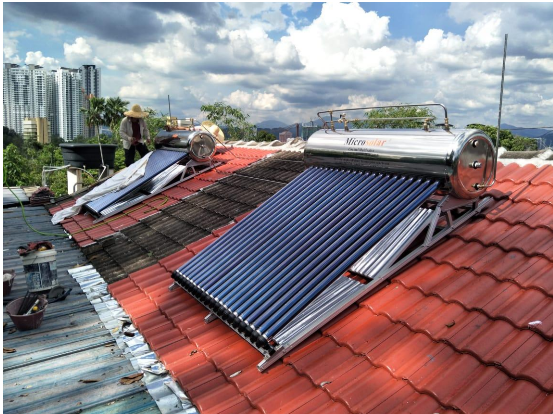
2 units Microsolar Water Heater M60VTHE and 1 unit Microsolar Cooler at Kenny Hills Bukit Tunku Kuala Lumpur Malaysia 2021
