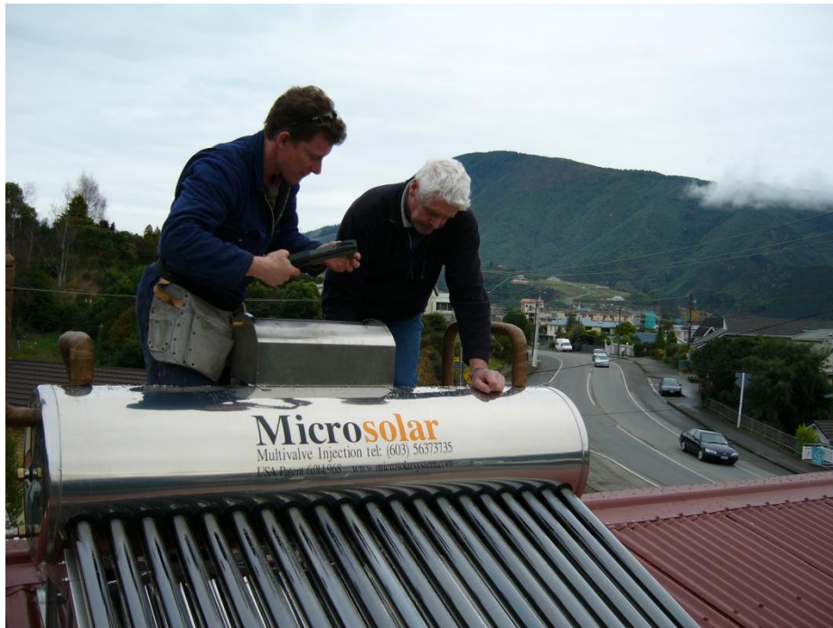
NZ Microsolar Distributor Vince Cowie installing Microsolar M60VTHE At Picton Marina, South Island New Zealand.
