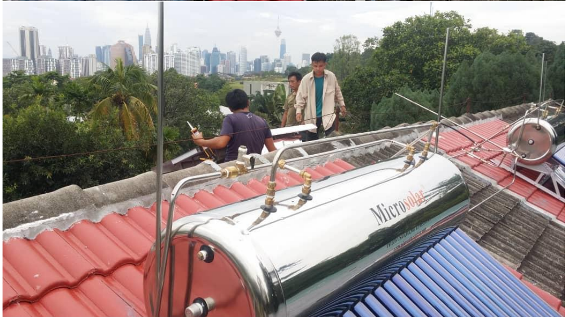
Installing 2 units Microsolar Water Heaters and 1 unit Microsolar Cooler at Kenny Hills Kuala Lumpur Malaysia 2021.
