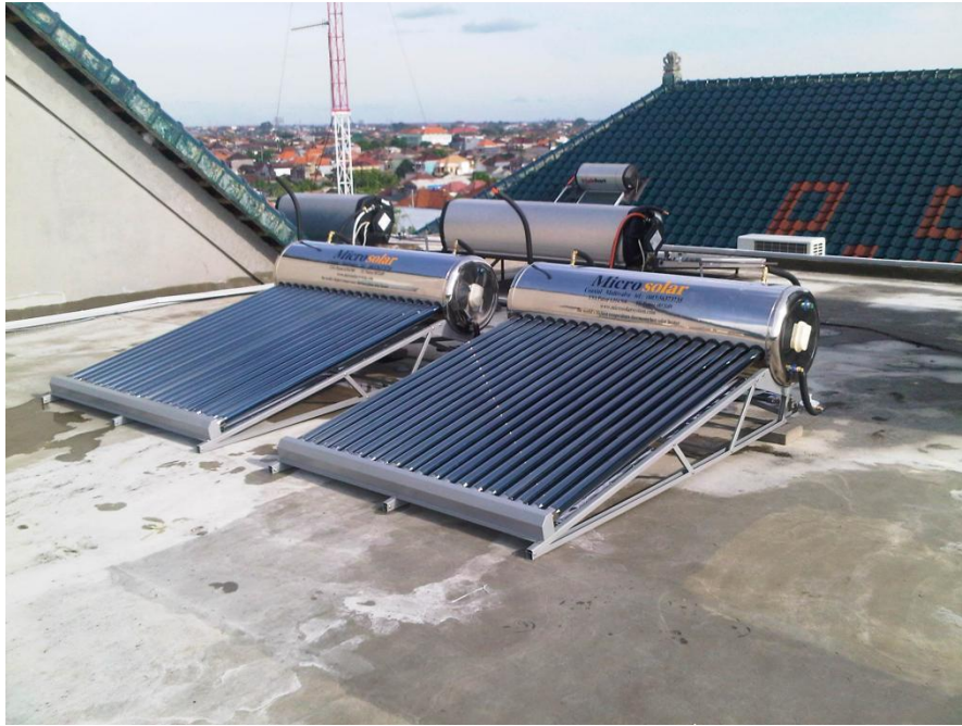
Microsolar M80VTHE Water Heaters installed at Bali Med Hospital Denpasar Bali Indonesia 2010
