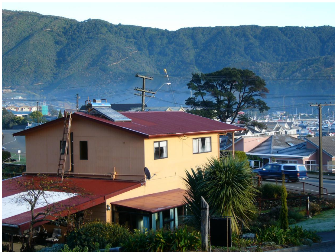
Microsolar Heater M60VTHE installed near Picton Marina, South Island New Zealand.
