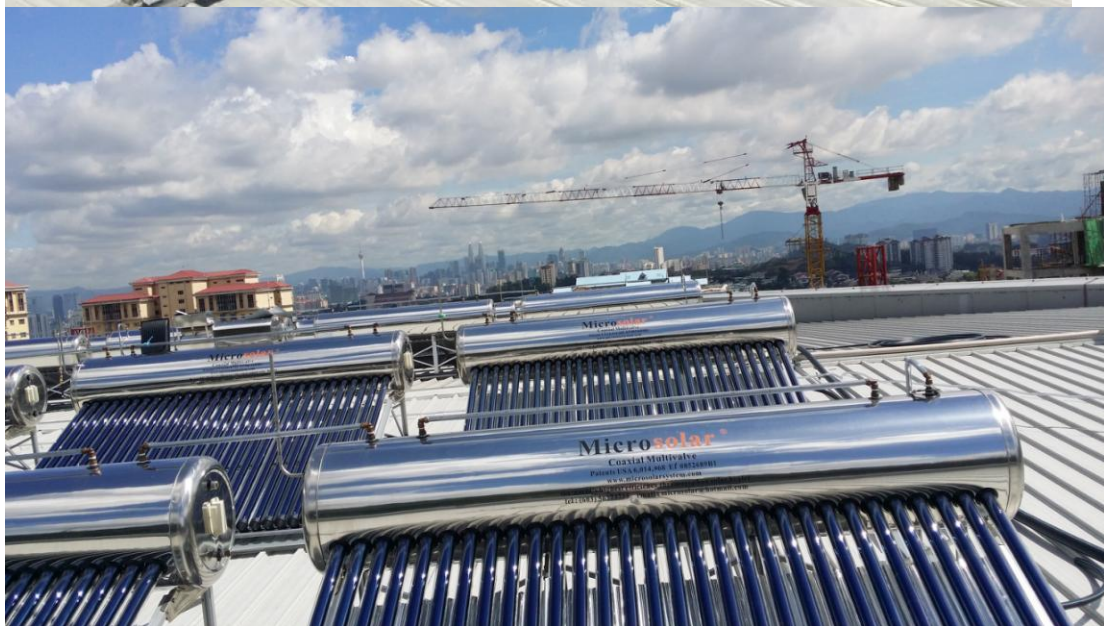
50 units Microsolar Water Heaters M80VTHE at University Campus and Hotel at Taman Connaught Cheras Kuala Lumpur Malaysia 2017 Ar Teoh Siang Teik discussion with installation team
